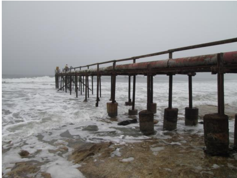
Figure 5: Existing seawater abstraction jetty for the Salt Works
